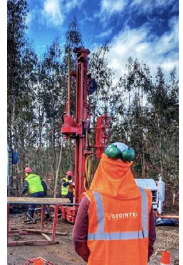
CAP04 FULL GEOTECHNICAL ASSESSMENT
